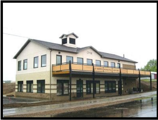
AIRPORT ADMINISTRATION BUILDING
