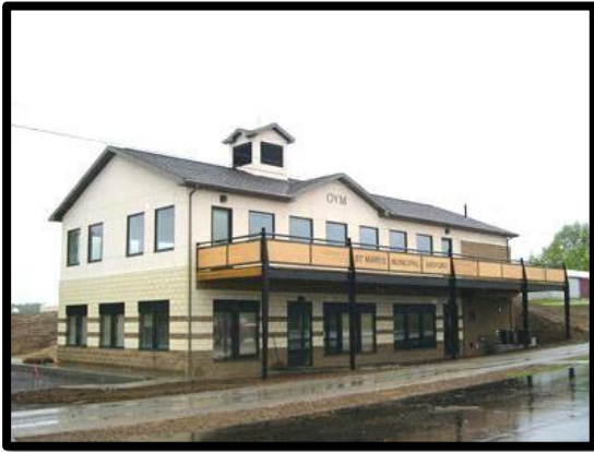
AIRPORT ADMINISTRATION BUILDING
