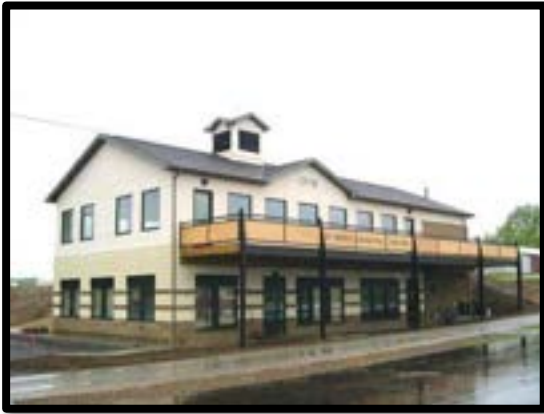
AIRPORT ADMINISTRATION BUILDING
